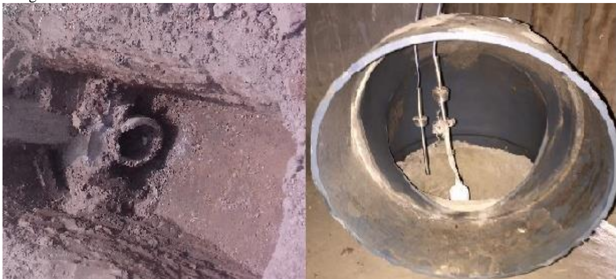
Fig -2 The inlet of the buried pipes where the blower is connected and outlet of the pipe in the tested room with temperature sensors connected to the pipe.
