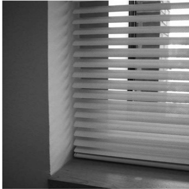
Figure 8: Venetian Blinds: Interior shading devices manually controlled[13].
